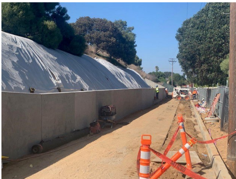
Diamond Street Bike Path Project 75% complete
